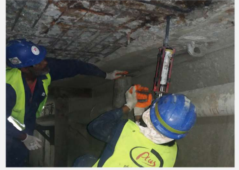
ANCHORING STEEL
