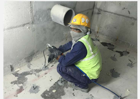
INJECTING CONCRETE
