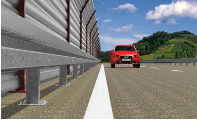
Sound insulation walls
